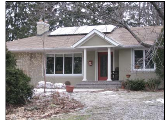
(Above: 2.27 kW Photovoltaic system, installed December 2008 in Oakville.)
